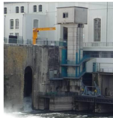
Pic. 28 : The fish lift at Tuilières
